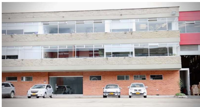
Figura No. 3 Entrada Bodega No. 11 – AEPI – Edexa S.A.S.
